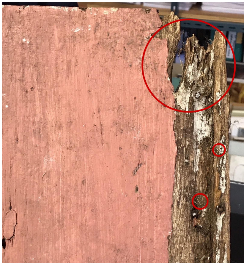
Figure 11: Traces of pine tree leaves left in the joints of the canopy can be seen in the wood.
